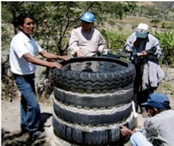
Alfonso (left) explains how to make a rainwater harvesting tank with used tires.
