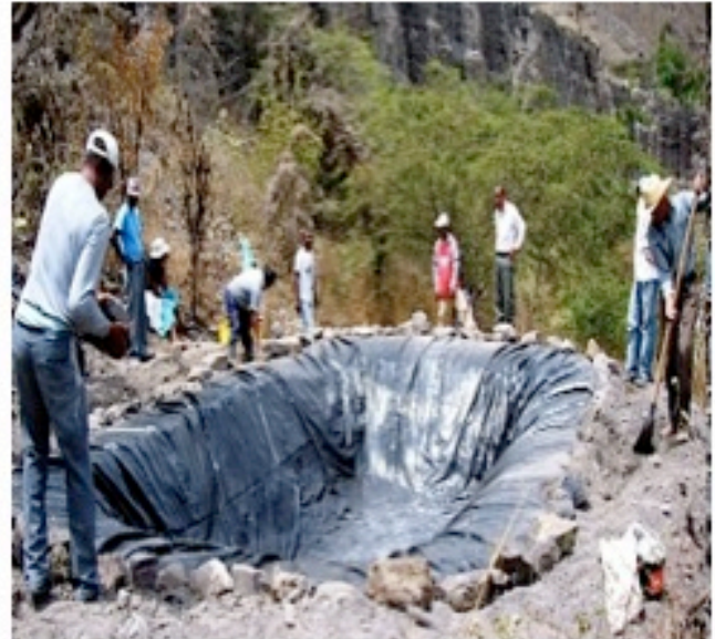
A "minga", or community work day in Quichua is organized to prepare a storage pond.
